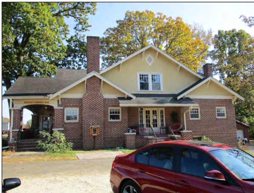
Photograph 4: Northwest elevation of 10233 N. Main St.; looking southeast. (2016)
