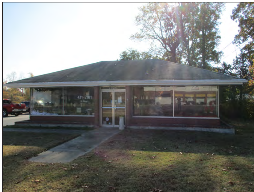
Photograph 10: Façade (northeast elevation) of 10219 N. Main St.; looking southwest. (2016)
