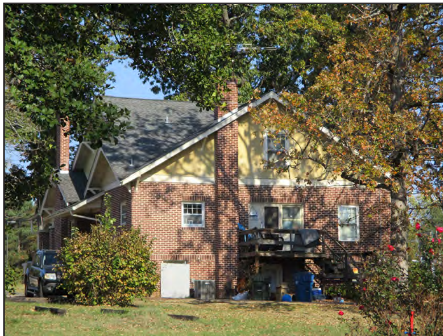
Photograph 5: Rear (southwest) elevation of 10233 N. Main St; looking northeast. (2016)
