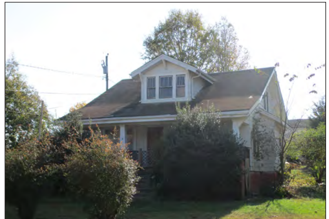
Photograph 16: Façade of 10320 S Main St.; looking southwest (2016)
