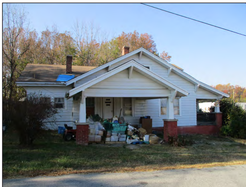
Photograph 17: Oblique view of 10320 S Main St.; looking northwest. (2016)
