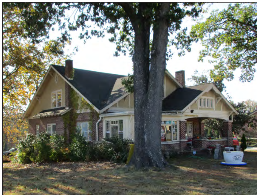
Photograph 6: Oblique view of facade and southeast elevation.; looking southwest. (2016)
