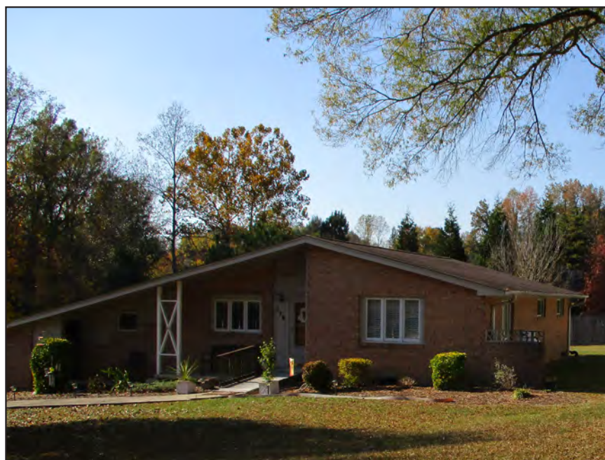
Photograph 14: Oblique view of 110 Marshall St.; looking west. (2016)
