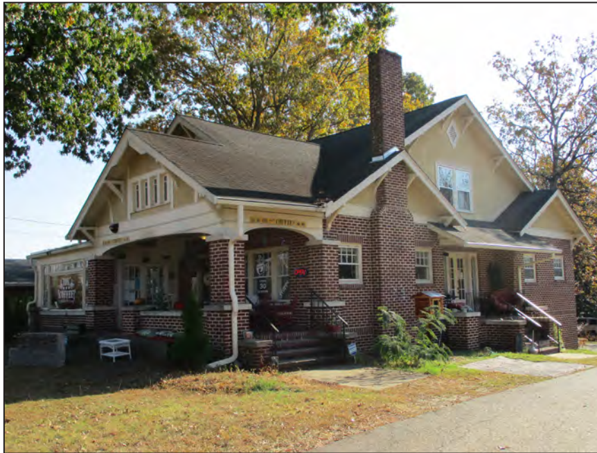
Photograph 3: Northwest elevation of 10233 N. Main St.; looking southeast. (2016)
