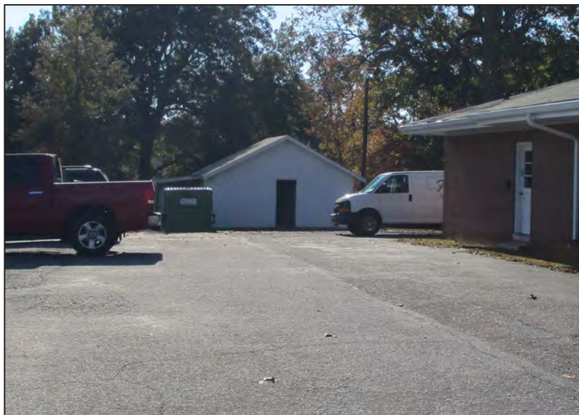
Photograph 12: Shed at 10233 N. Main St.; looking southwest. (2016)
